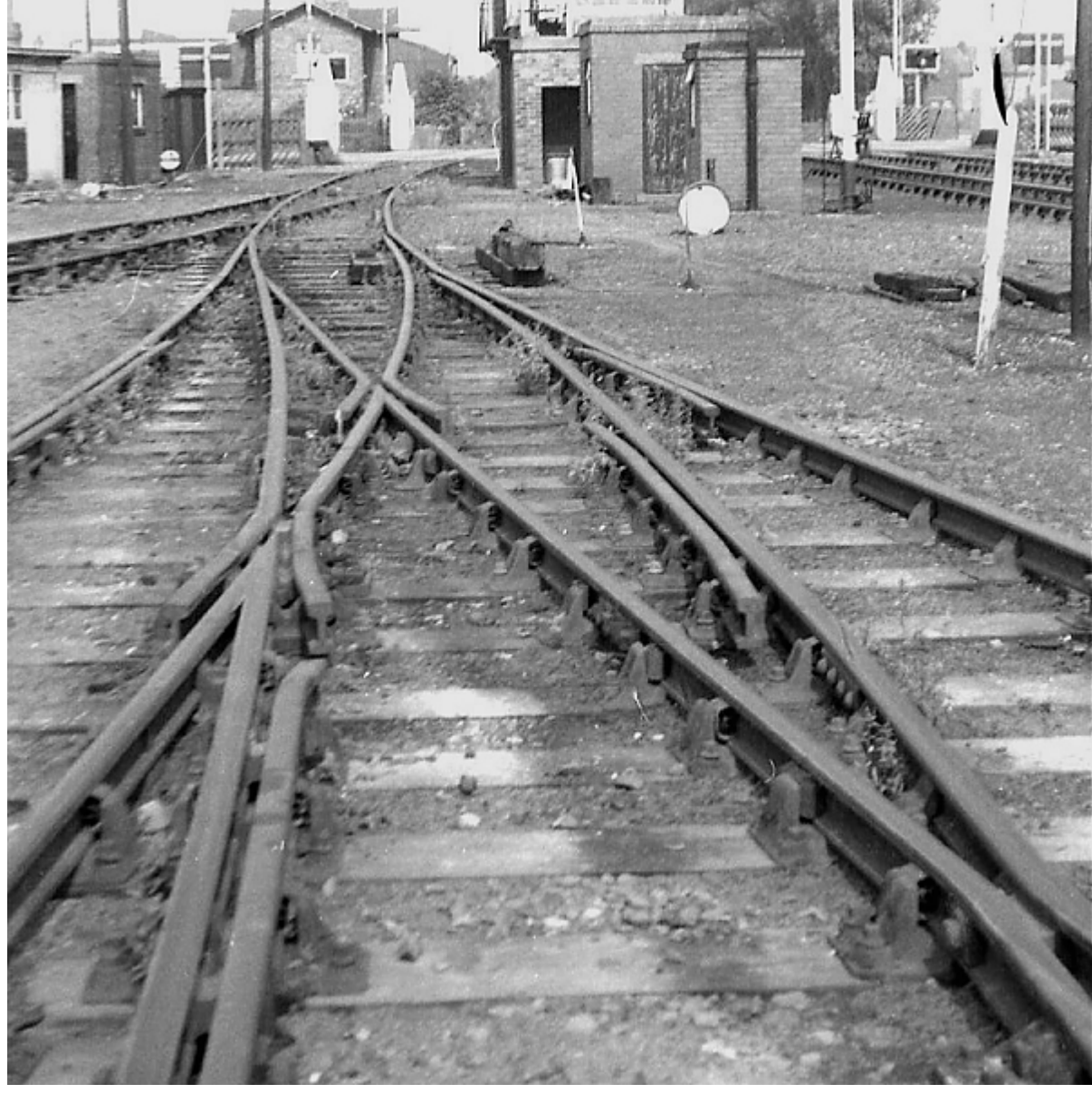
A type 2 tandem turnout (thanks to Mick Nicholson for the photo)
